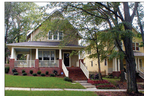
Infill housing can take many forms, but one should consider the local architecture and scale in a given area of the neighborhood.
