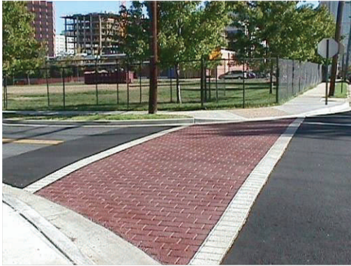
Textured brick and pavement, like the crosswalk shown above in Arlington, Virginia, can increase awareness of pedestrians.
