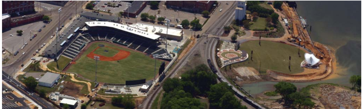
Aerial view of the new Riverwalk Stadium and Riverwalk Amphitheatre
