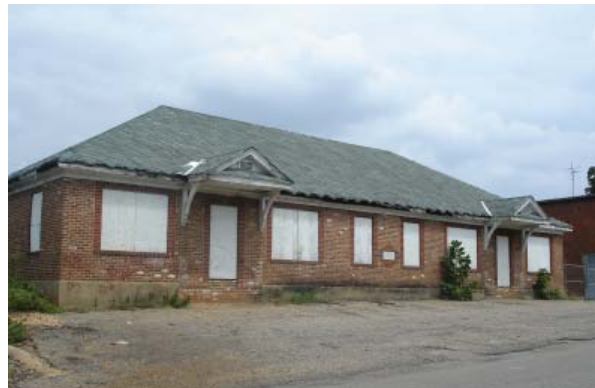
At risk frontage
