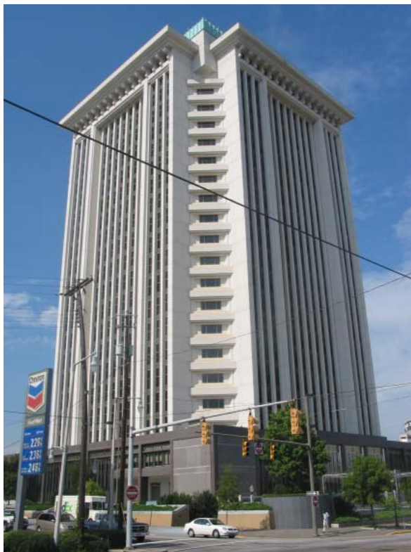
The RSA Tower
