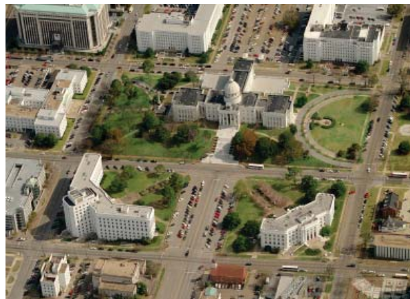
The Capitol Complex, current conditions
