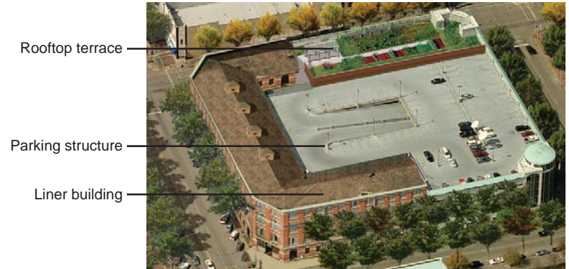
Garage wrapped with multi-story habitable space
