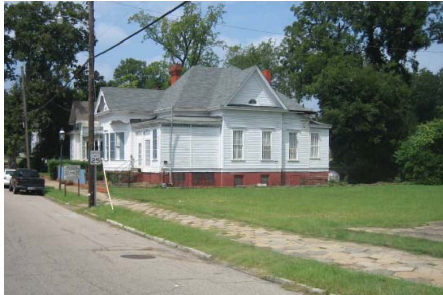
Before: A neighborhood street in Cottage Hill, existing conditions
