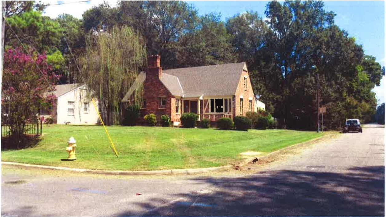
Before partial vinyl window replacement
