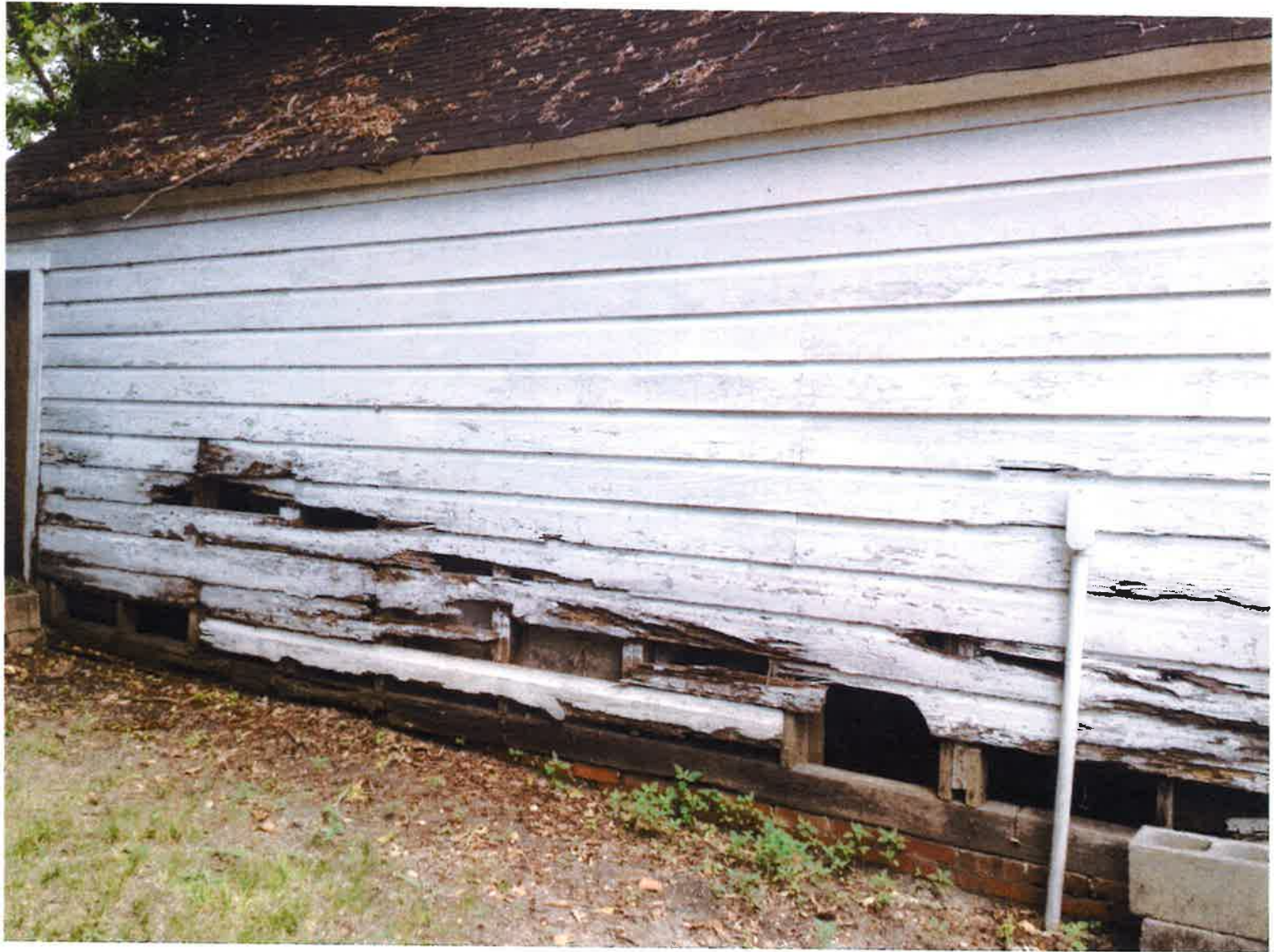
Badly rotted wood on detached garage...exact same shingles will be used for new garage
