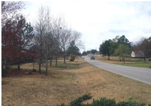
Low-density residential street with vegetated open channel
