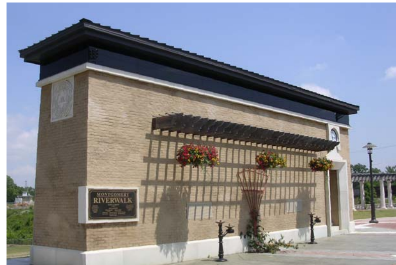
Monument at Riverwalk Park
